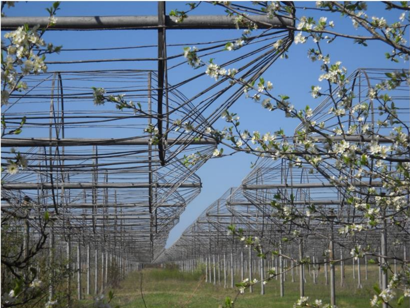
The world's largest UTR-2 radio telescope (N-S arm, 1.9 km x 60 m) Frequency range - 8... 32 MHz; number of elements - 2040; effective area - 150,000 square meters.
