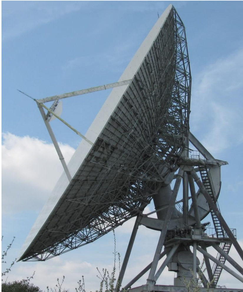
Antenna MARK-4B and BWG system
